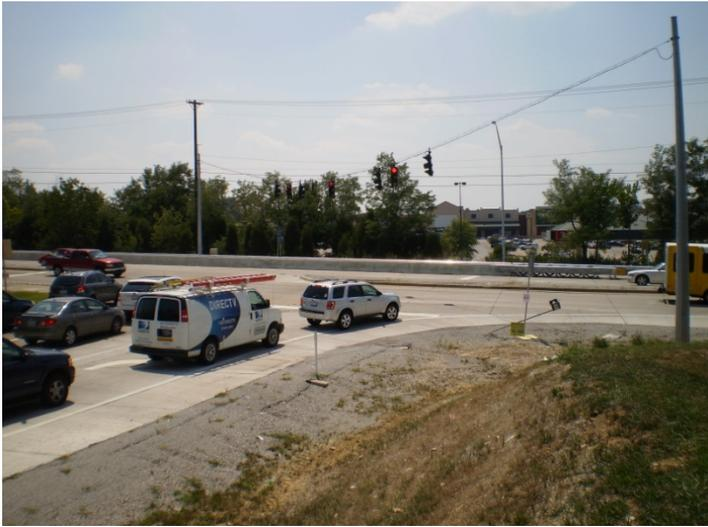
**View of ramp widened at the intersection with US 31E and beginning section of concrete barrier with crash cushion (Looking west)**
